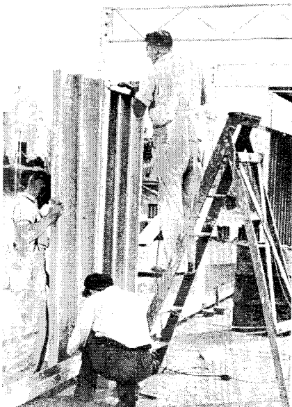
STEEL LOCK PANEL ASSEMBLY
